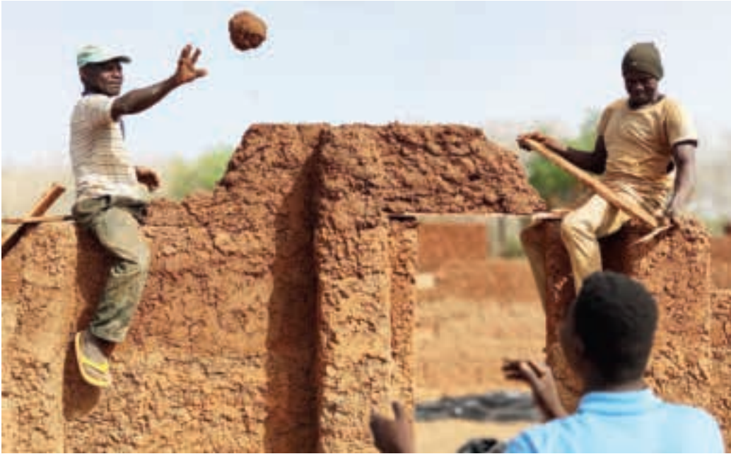
Educational Training Campus in Tatale, Ghana (ongoing)
