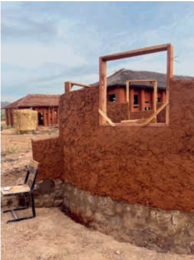
Educational Training Campus in Tatale, Ghana (ongoing)
