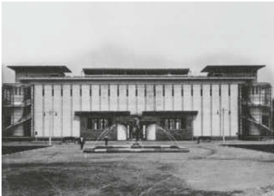
The office building for the pattern factory designed by Walter Gropius and his partner Adolf Meyer, with side stairwells entirely of glass, at the Deutscher Werkbund exhibition in Cologne, 1914.
