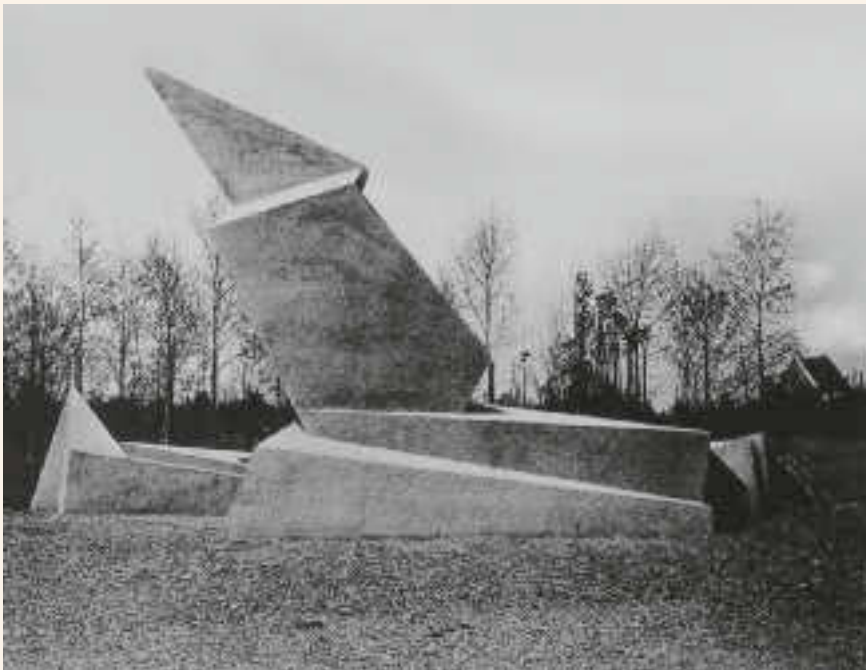
This memorial to the workers murdered in the Kapp Putsch of March 1920, built in 1922 to a design by Walter Gropius at the Cemetery of Honor in Weimar, is distinguished by its Expressionist language of forms.
